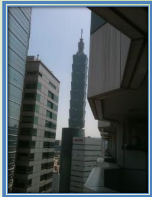
This is the second highest building in the world ... called Taipei 101
