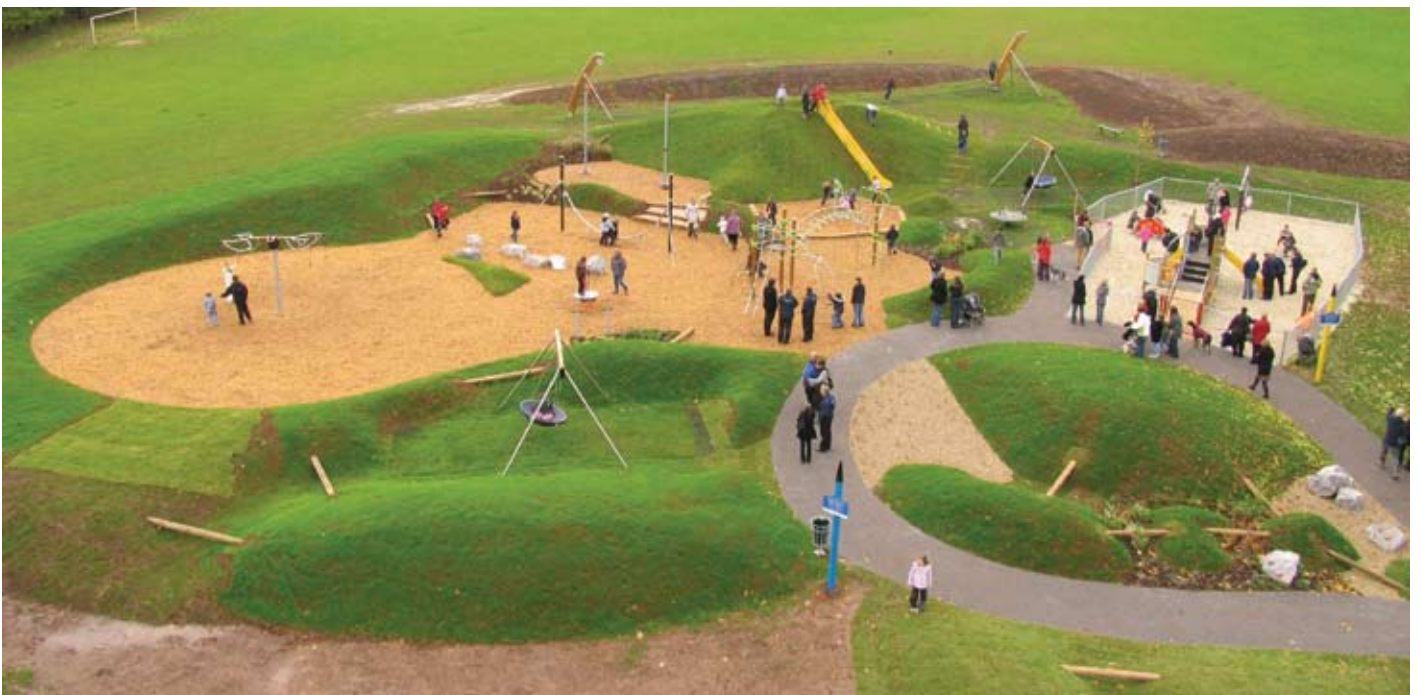
A completed Playbuilder site in Taunton Deane, Somerset. Photo provided by Proludic
